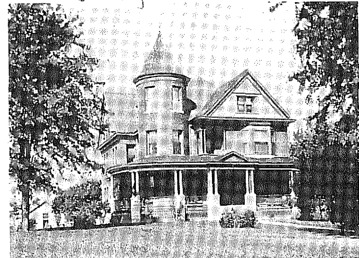
Dr. and Mrs. Still's new home on Osteopathy Street, completed 1899
