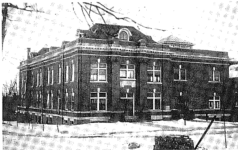
ASO Hospital on the corner of Jefferson and Osteopathy Streets, built 1905
